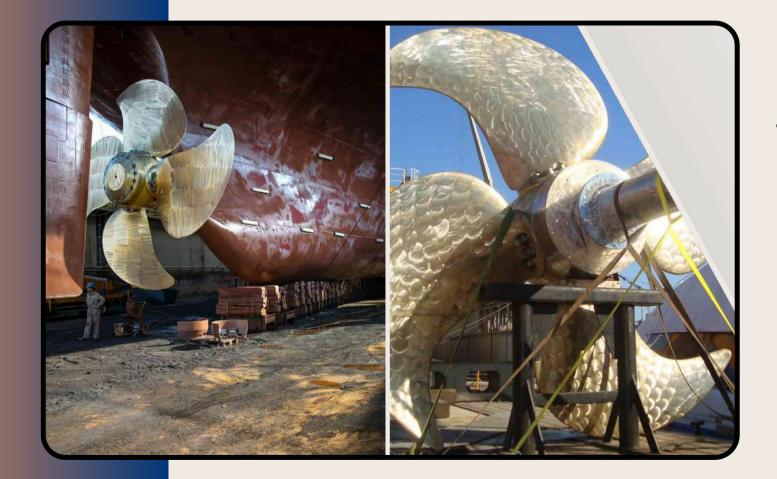
Repairing & maintenance and renewal following work items: -Dismantling and refitting of shaft coupling -Withdrawal and fitting back of the shaft -Dismantling and refitting of intermediate shaft -Dismantling and refitting of fix propeller -Dismantling and refitting of CPP propeller blades -Renewal of simplex seals
